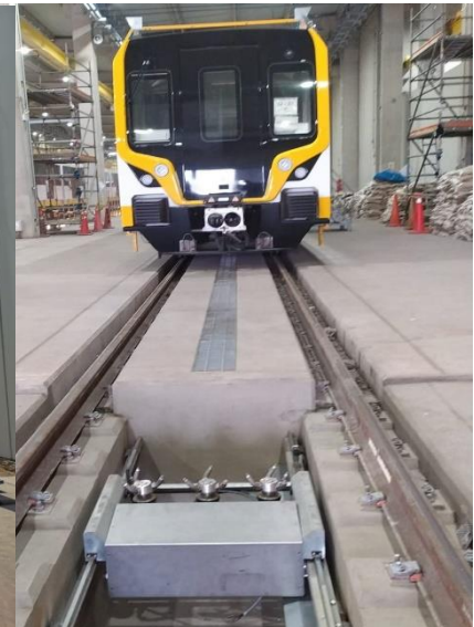
Underframe Washing at Lima (Peru)
